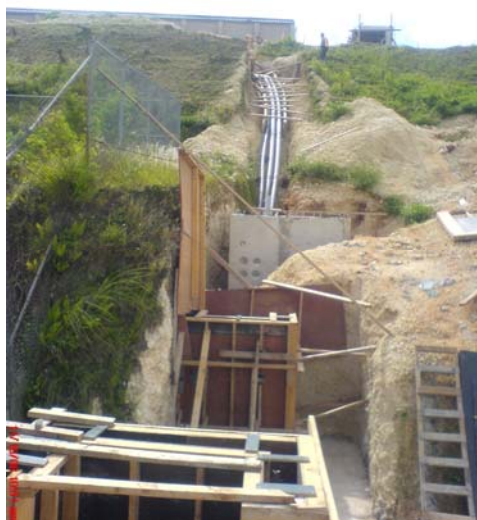
Macheche – GAA 34.5 kV UG - CONSTRUCTION
