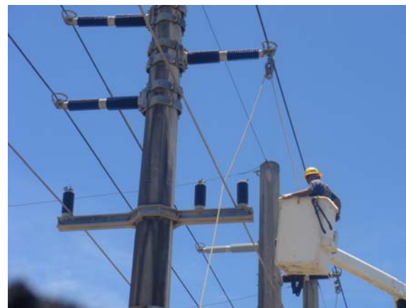
Harmon to GIAT Reconductoring - COMPLETED
