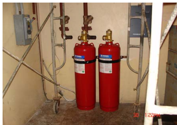
Fire Protection Upgrade at Dededo CT - CONSTRUCTION
