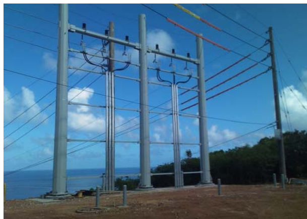
Harmon to Tanguisson – 34.5 KV UG - CONSTRUCTION
