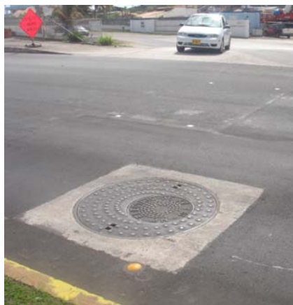
Harmon to Tumon 34.5 kV UG - COMPLETED
