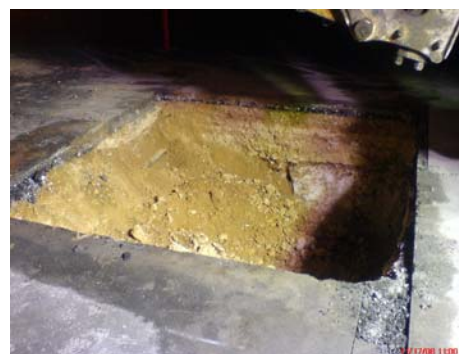
San Vitores to Macheche 34.5 kV UG - CONSTRUCTION
