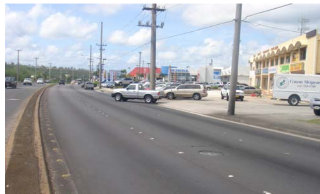
Tamuning to Tumon 34.5 kV UG - COMPLETED
